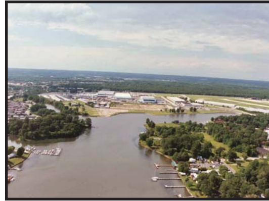
Martin State was the home of the Glenn L. Martin aircraft factory. Your seaplane will be moored in the lagoon where the China Clippers were launched 60 years ago. Note the paved runway to the right of the factory.
