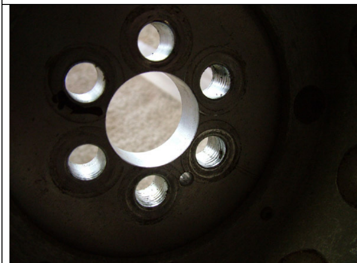
Thread marks are visible in the flywheel holes consistent with fretting. All three flywheels had these imprints.
